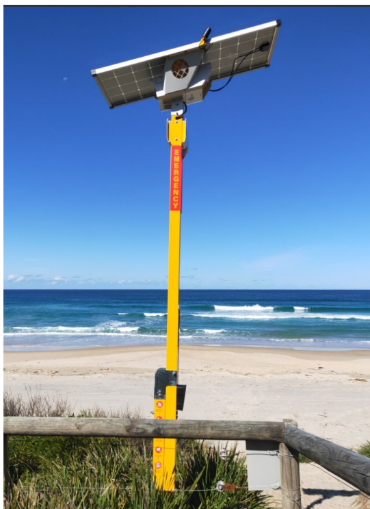
Figure 5 Racecourse Beach recently installed AUG 25.
