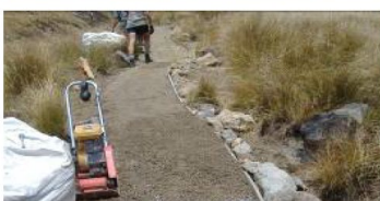
Figure 58 – With the geocells filled the walking surface can be applied and compacted
