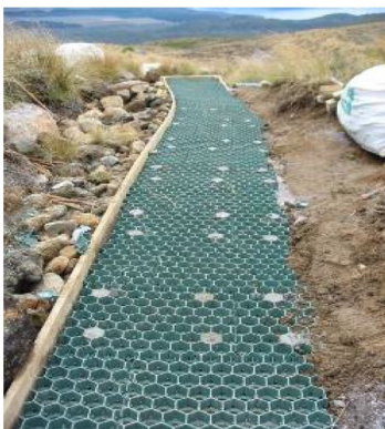
Figure 57 – To hold the cells in place a 12 mm reinforcing rod is driven into the soil. The individual cells containing the rods are then filled with a hardener to secure the geocells in place.
